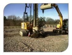
The Dudley site was geotechnically very difficult due to old mine works leaving varying rock profile and strata material. Significant site probing was required, along with profiling of the rock levels to give strength of material. Grout stabilisation of mine workings had to be undertaken prior to piling to mitigate settlement and subsidence; the pile schedule was then prepared based on the grouting records.
