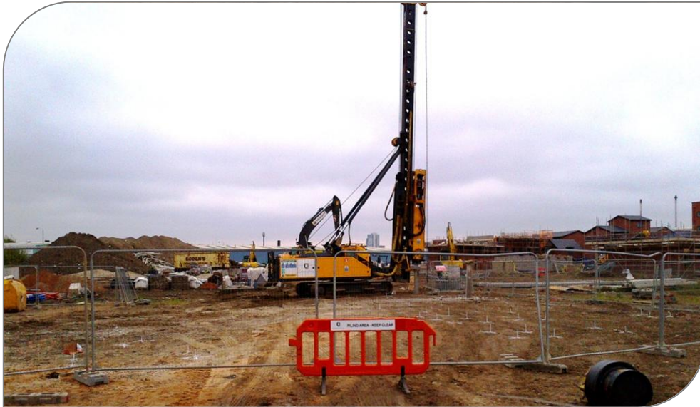
Image shown is of piling works at Yarn Street, Hunslett
