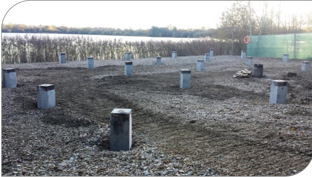
Image shown is of piles installed at Longdales, Lechlade
