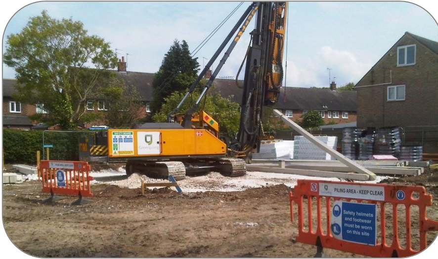
Image shown is of pre-cast piling at Rokeby Avenue, Hull
