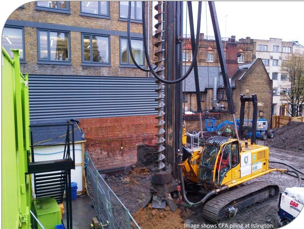
Image shows CFA piling at Islington
