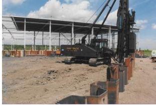
Image of Green Piling's first rig completing our first ever project
